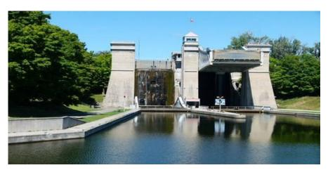
Near the museum are the Peterborough Lift Locks. Opened in 1904 and designated as a Canadian National Historic Site, this is the highest hydraulic lift lock in the world. Powered by gravity, the Lift Lock towers almost 20 m (65 ft) above the Trent Canal, enabling lifts in two counter-balanced, bath-tub-like chambers. The locks can be visited, and a 2-hour sightseeing cruise is available as well.
